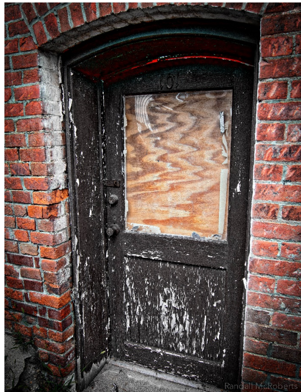
Basement Door: Randy McRoberts – Creative Commons
